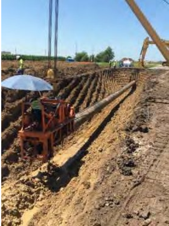
Photo 7: Conventional bore under a roadway
