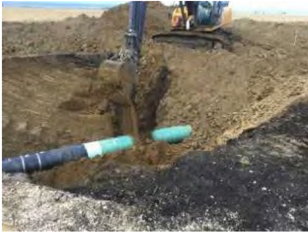
Photo 12: Subsoil being used to backfill the ditch line
