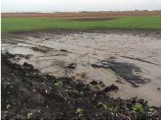
Photo 3: Impacts of improper dewatering practices
