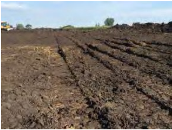
Photo 1: Stripping topsoil in wet conditions may cause soil mixing
