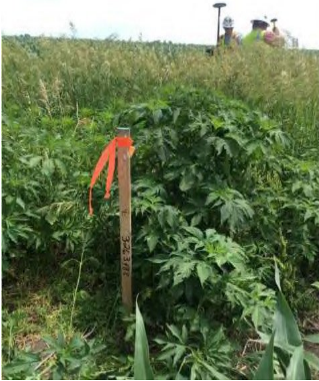
Photo 5: Right-of-way staking
