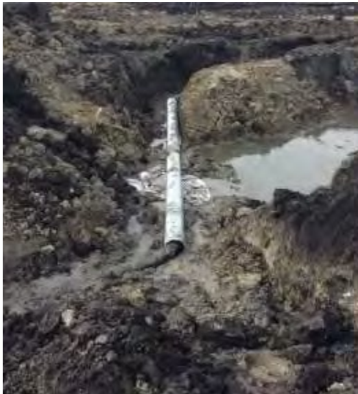
Photo 12: The original alignment of the tile has been altered to cross the ditch line at a more favorable angle
