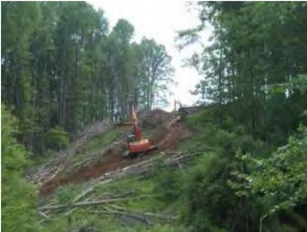
Photo 6: Right-of-way clearing
