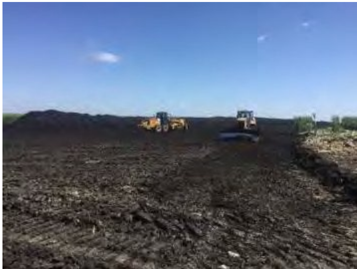
Photo 7: Topsoil removal and stockpiling
