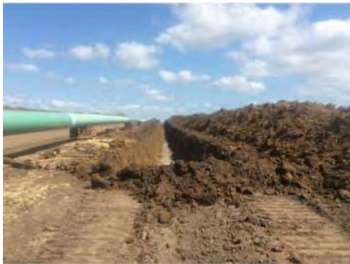
Photo 8: Trenching of the ditch line
