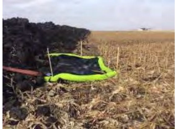
Photo 4: Using erosion logs as a secondary containment can greatly reduce the deposition of silts onto adjacent lands
