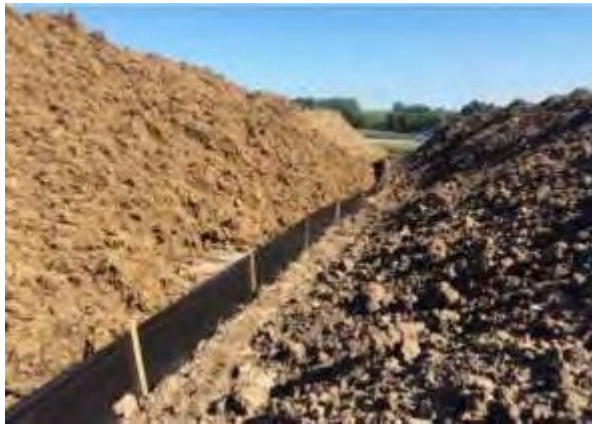
Photo 9: Proper separation of the topsoil and subsoil stockpiles
