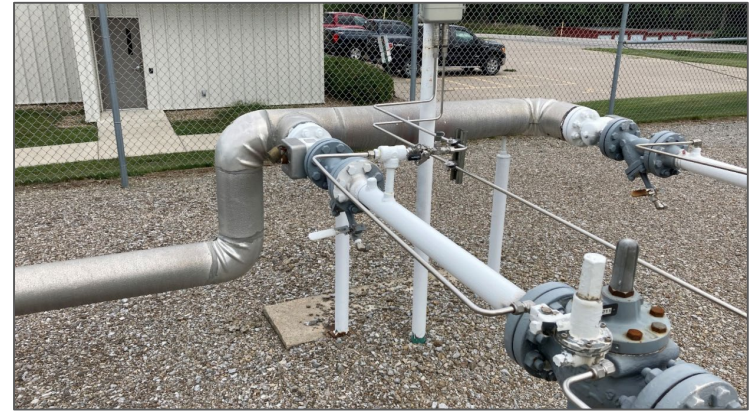
Inspect Under Insulation
