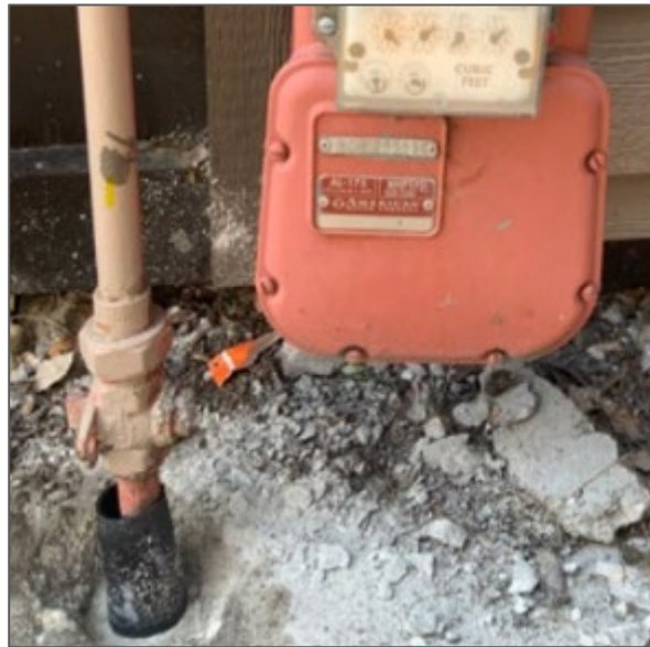
Inspect Soil-to-Air Interface?
