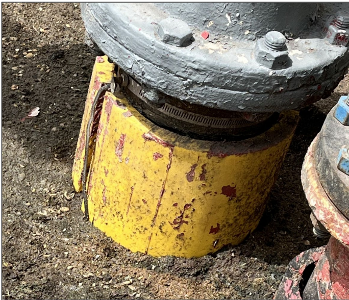
Inspect Soil-to-Air Interface?
