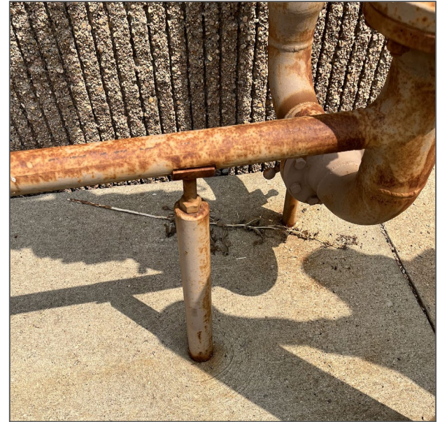
Example of Pipe Support
